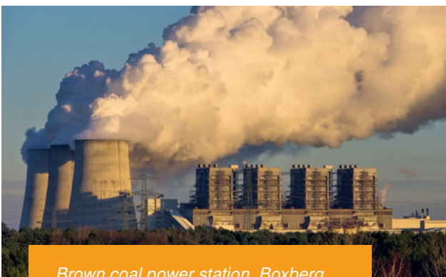
Brown coal power station, Boxberg
